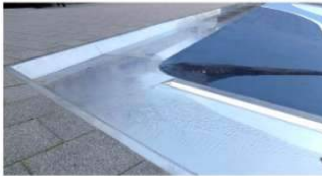
the "water wall" takes the water from further surroundings into the deep basin
