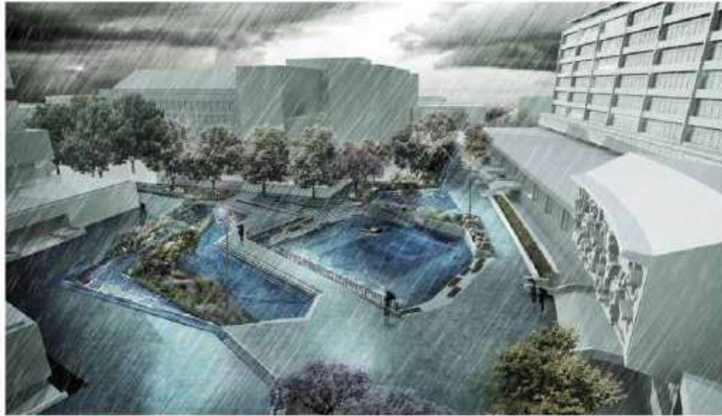
The Bentheimplein water square as temporary water storage facility, artist's impression of the scene during a downpour
